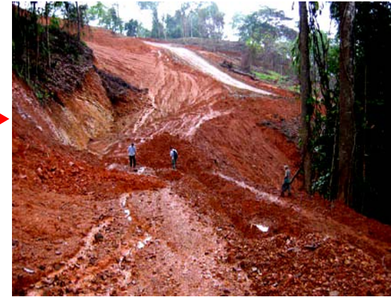
Soil and slopes erosion,
